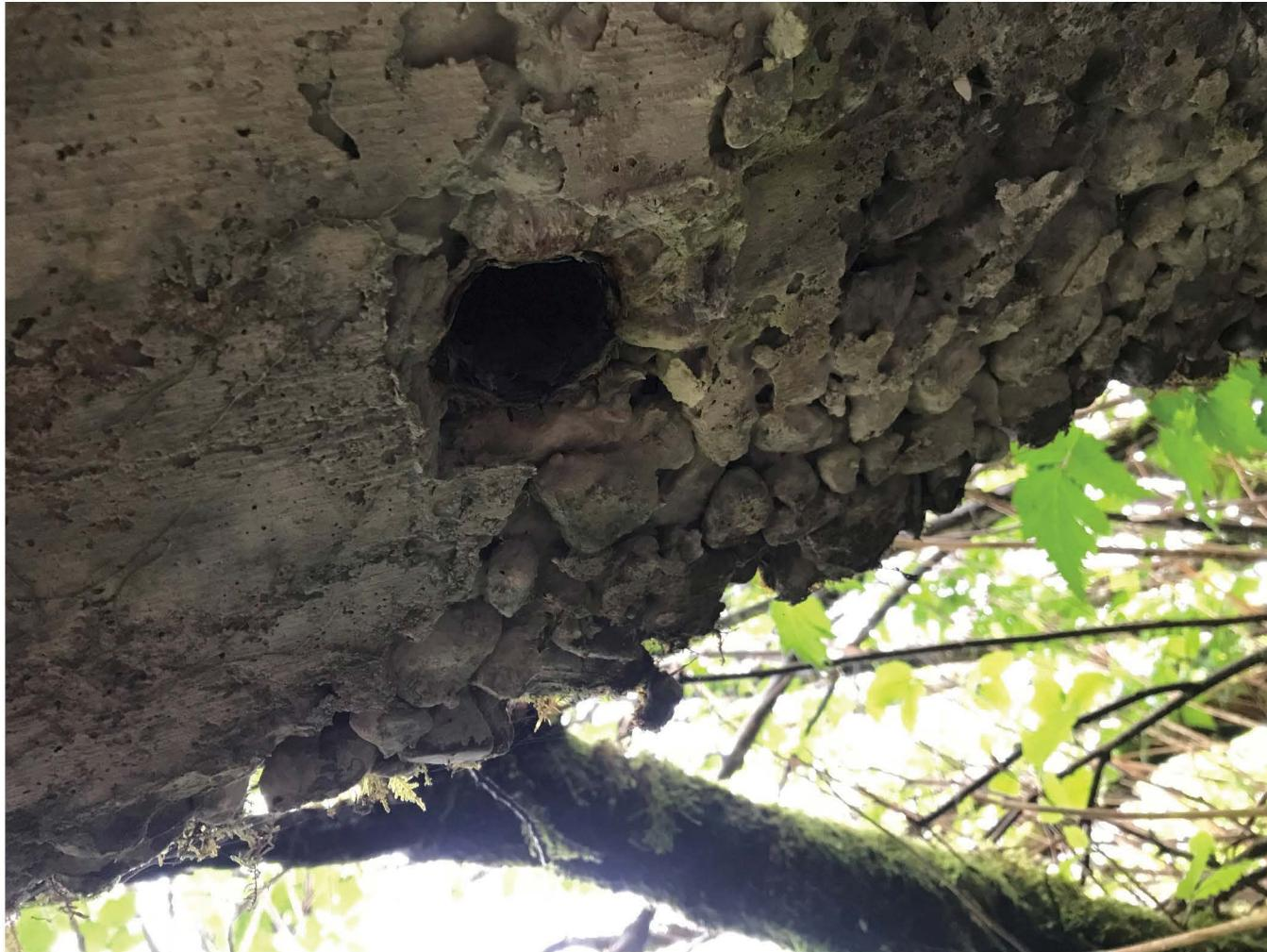
**Remains of Window Support, Spalling**
