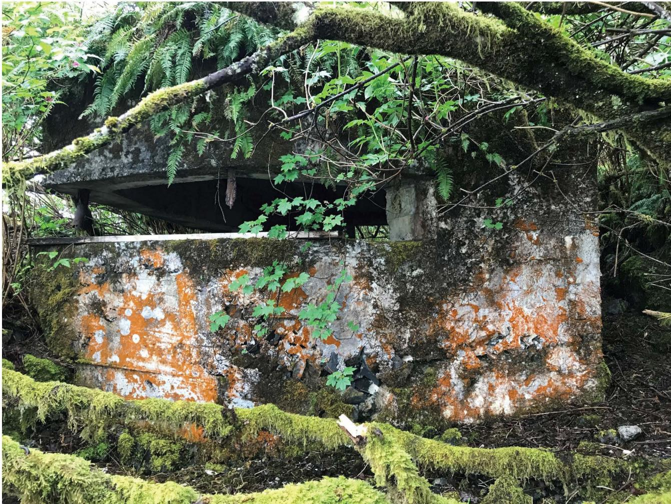
**Light Spalling on NW Exterior Wall**
